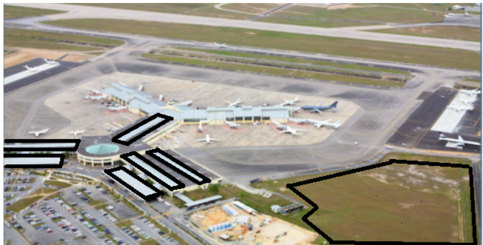
FIGURE 14 Location for Potential Installation of Solar Panels at POS Airport
